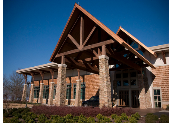
The lodge at Lake Guntersville State Park provides a comfortable stay for company functions.
